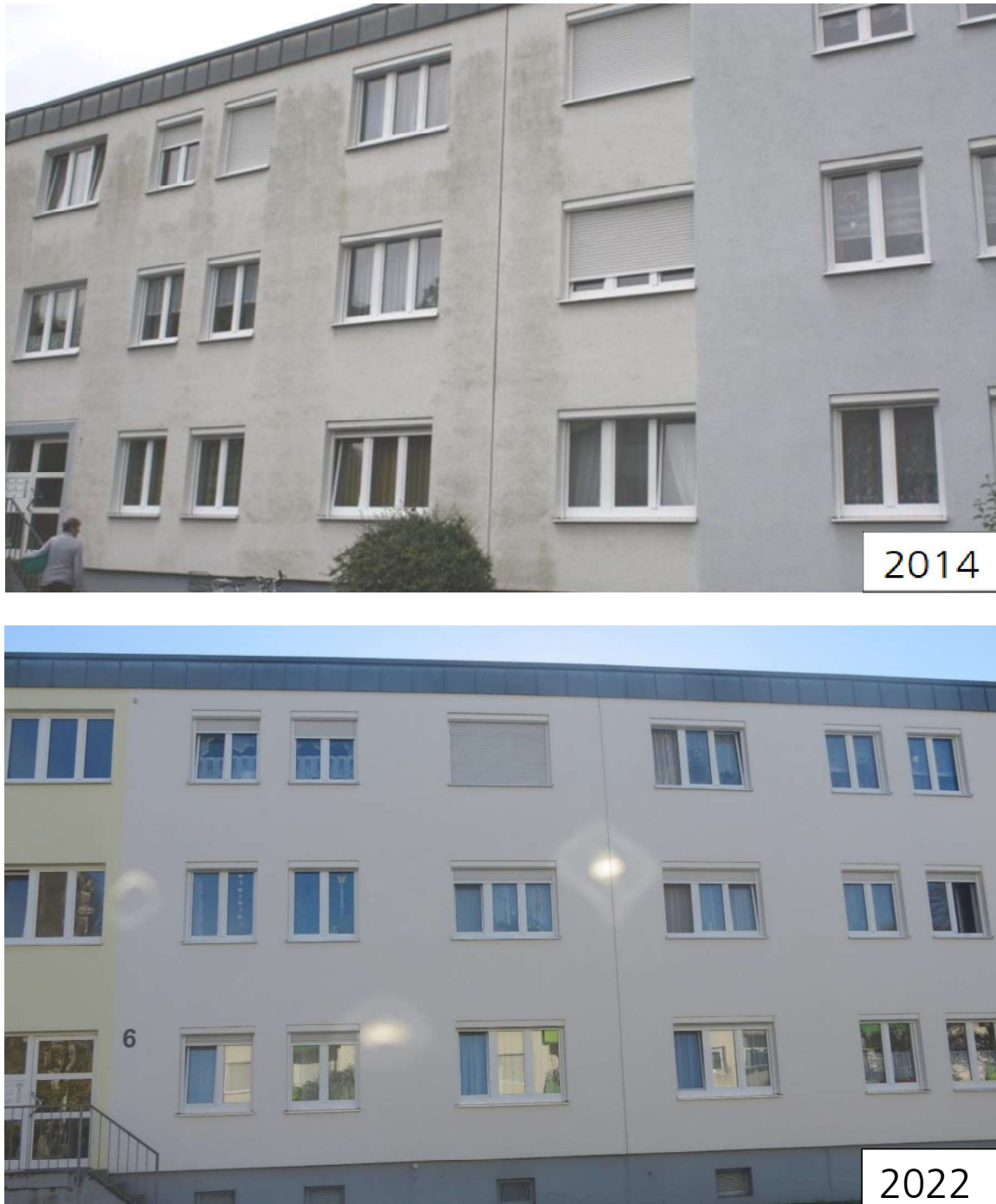
Figure 21: North façade of object 34, in 2014 (top) with noticeable discolorations of the white plaster surfaces and in 2022 (bottom), freshly painted approx. two years before.
