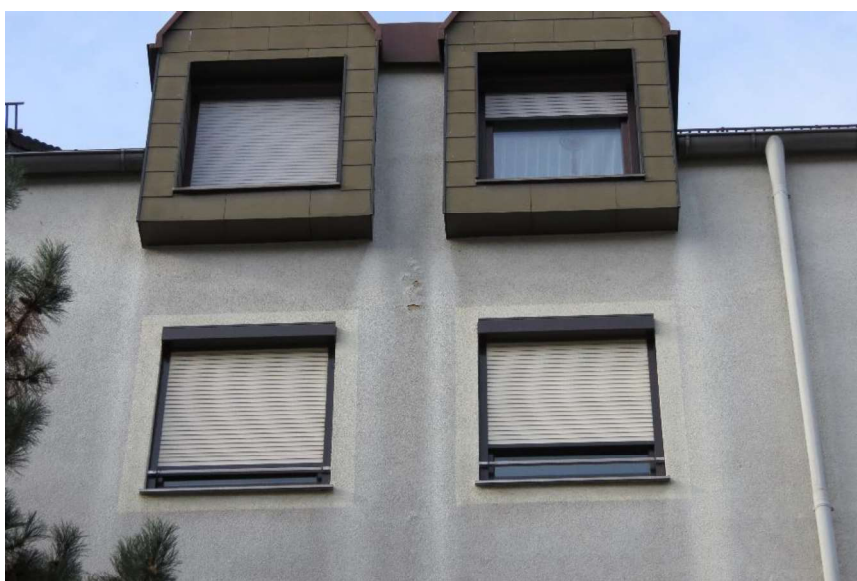
Figure 12: View of the east façade of the part of the residential complex that borders Mathildenstrasse. Noticeable crack formation and plaster separation between the windows.
