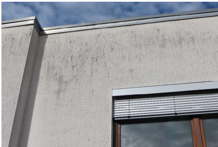
Figure 34: View of the upper south facade.
