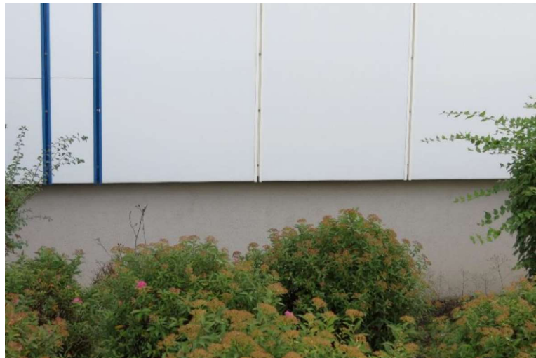
Figure 35: View of the base area of the north façade, which is insulated with purenotherm.
