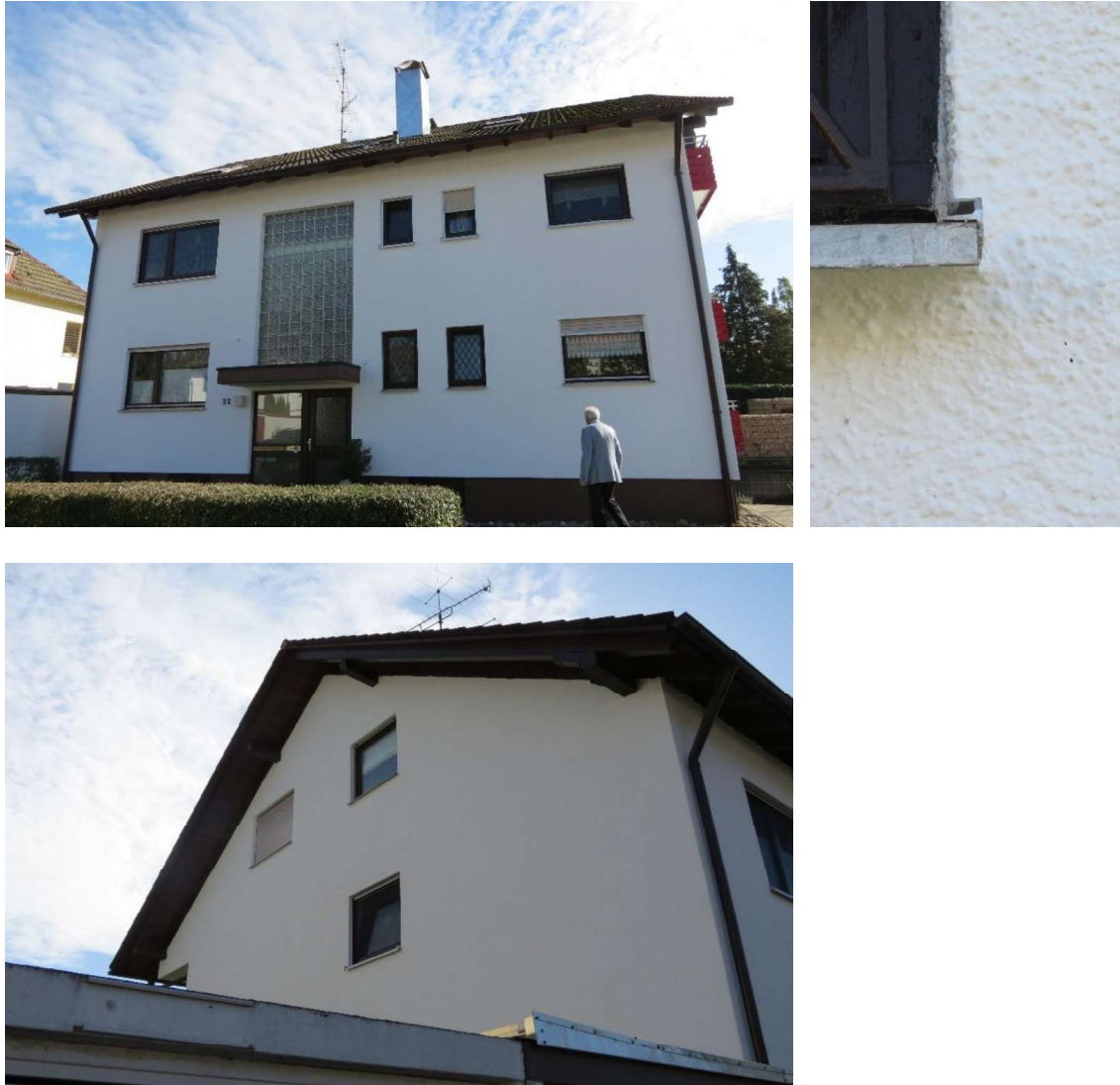
Figure 40: View of object 11 of the west (top left) and north façade (bottom) as well as a windowsill connection on the west side (top right).
