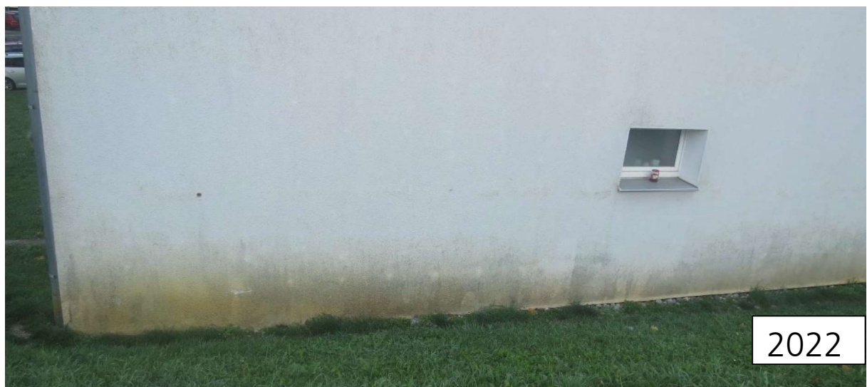
Figure 27: View of the lower east façade surface in 2014 (top) and 2022 (bottom) at the connection to the grass strips with noticeable algae growth and soiling of the plaster surface by spray water as well as the appearance of dowel areas.
