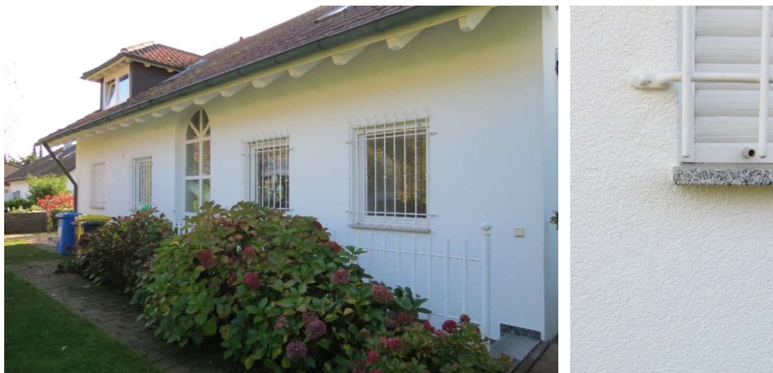
Figure 39: View of the north façade (left) and a windowsill connection (right) of object 4.
