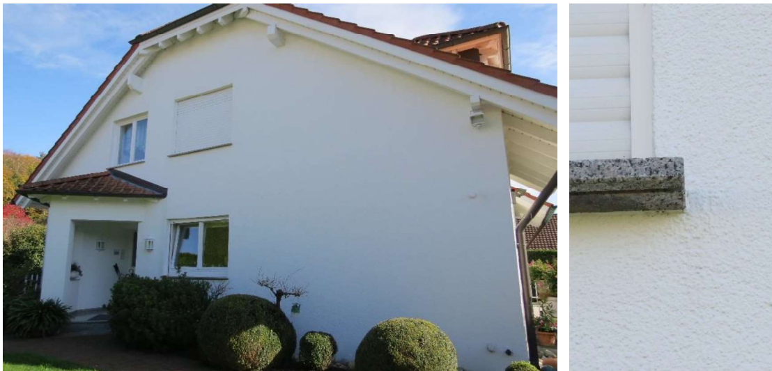
Figure 38: View of the west façade (left) and a windowsill connection (right) of object 4.
