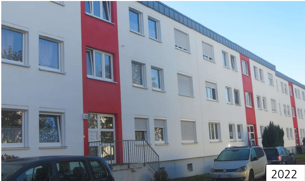
Figure 22: North view of object 33 (Bolzstr. 9–12, Geislingen a. d. Steige), in 2004 (top), 2014 (center) and 2022 (below).
