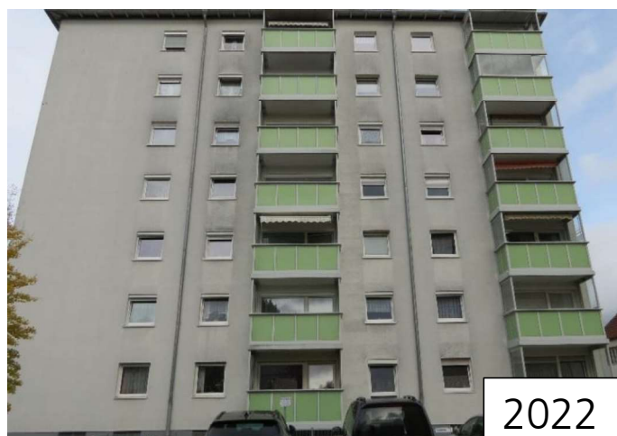
Figure 16: South view of the façade of object 56 (formerly Efastr.), in 2004 (top), 2014 (center) and 2022 (bottom).
