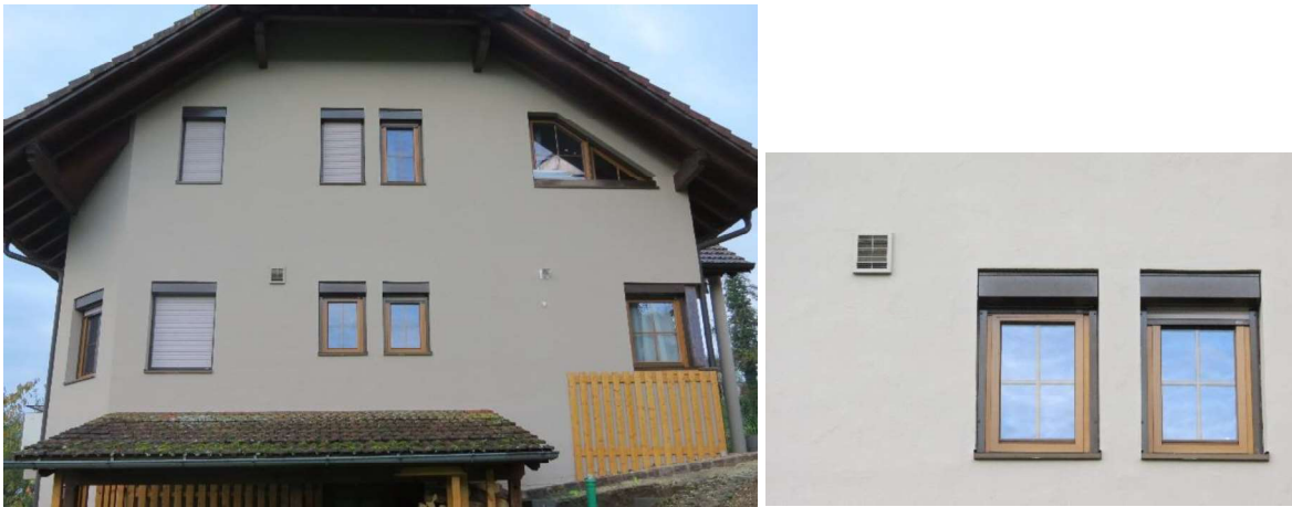
Figure 55: View of the north façade of object 9 with close-up of the ventilation opening next to the windows.
