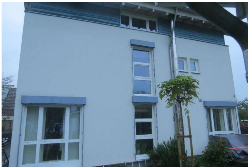
Figure 51: View of the south-west façade of object 9.
