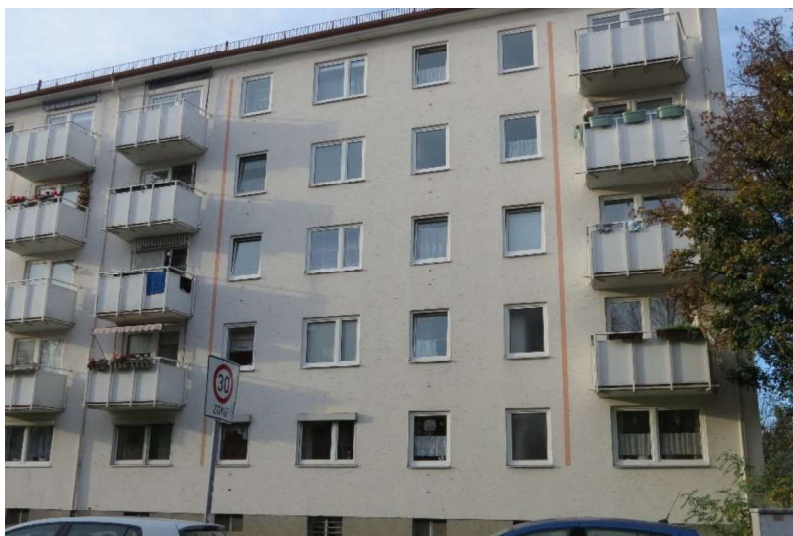
Figure 50: View of the north (top) and south façade (bottom) of object 8.
