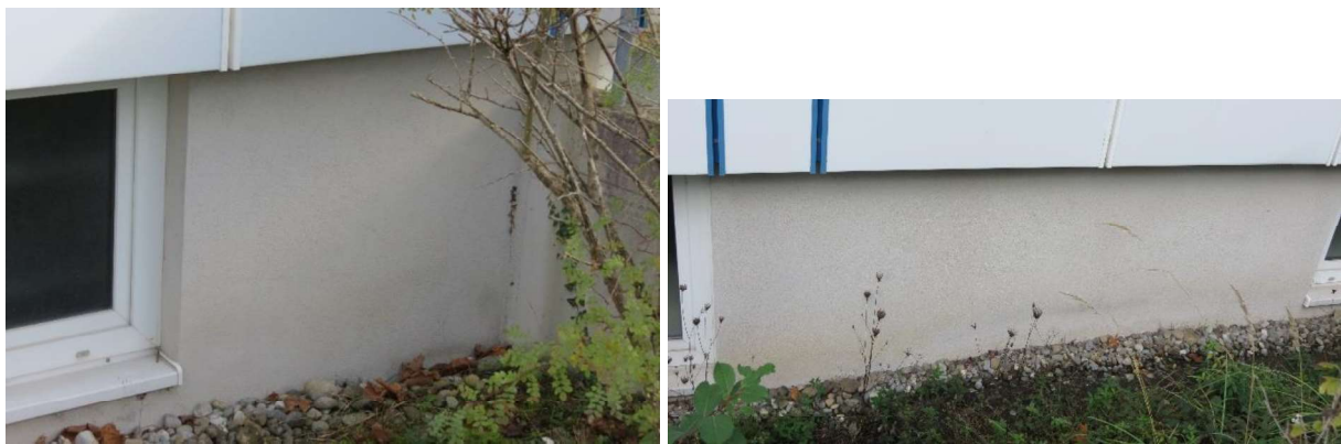
Figure 36: View of the base area of the west (left) and south (right) façade, which is insulated with purenotherm.
