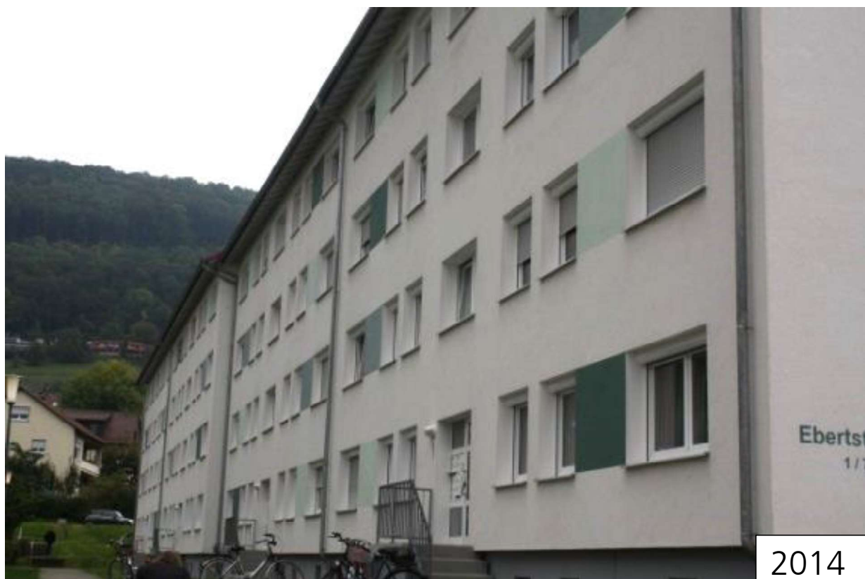
Figure 24: View of the north façade of property 32 (Ebertstr. 1–7, Geislingen a. d. Steige) in the period between 2004 and 2014.
