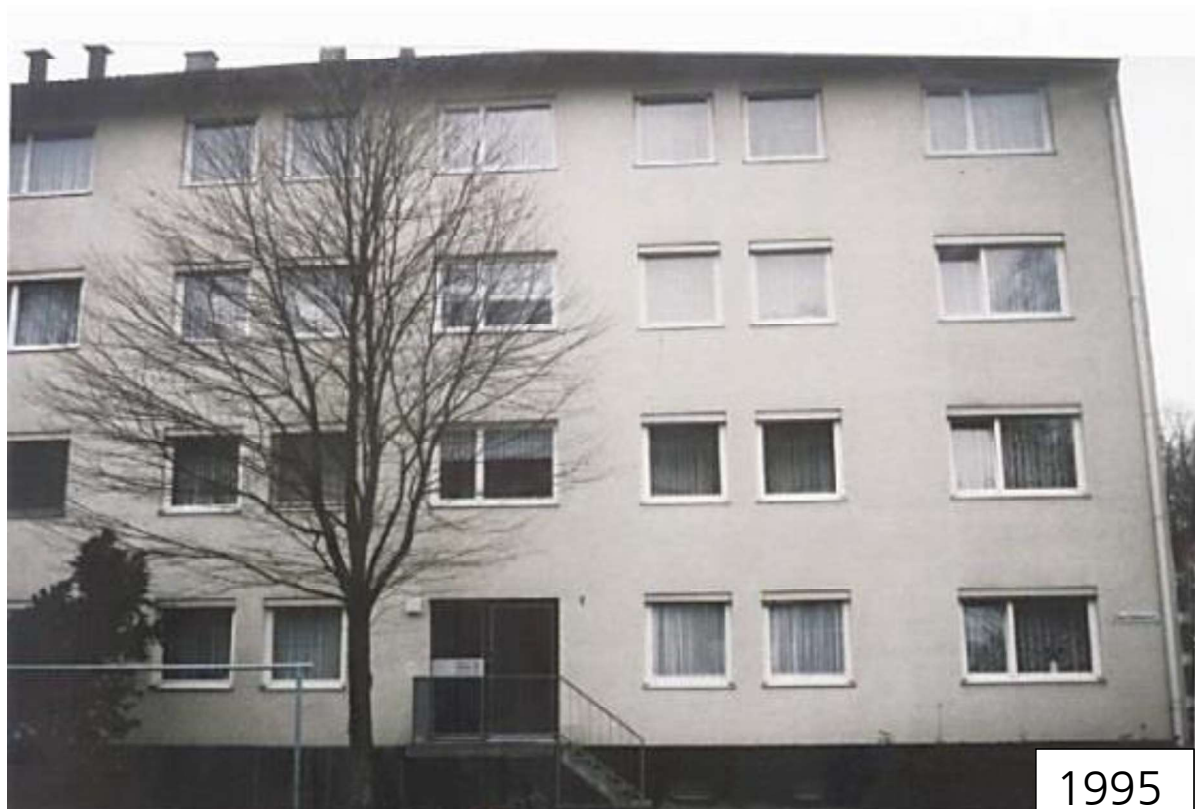
Figure 23: View of the north façade of property 32 (Ebertstr. 1–7, Geislingen a. d. Steige) in the period between 1983 and 1995.
