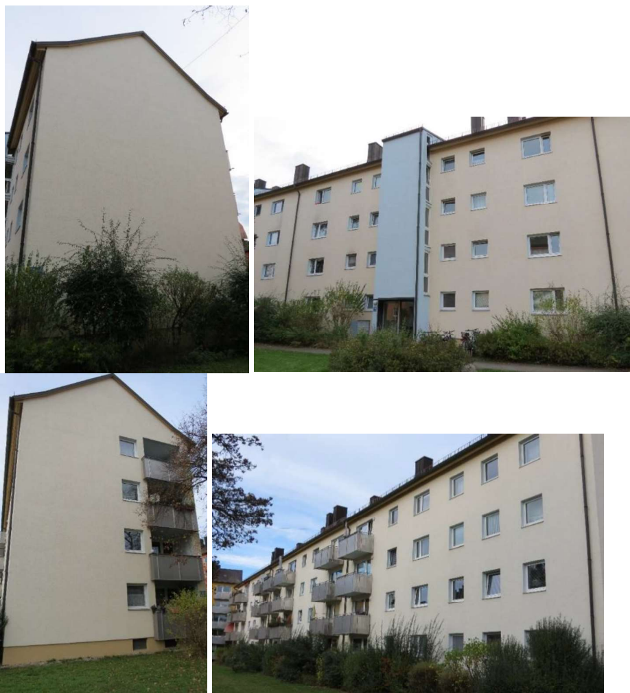
Figure 47: Views of the facades of house numbers 79–83. Top left: north façade. Top right: east façade. Bottom left: south façade. Bottom right: west façade.
