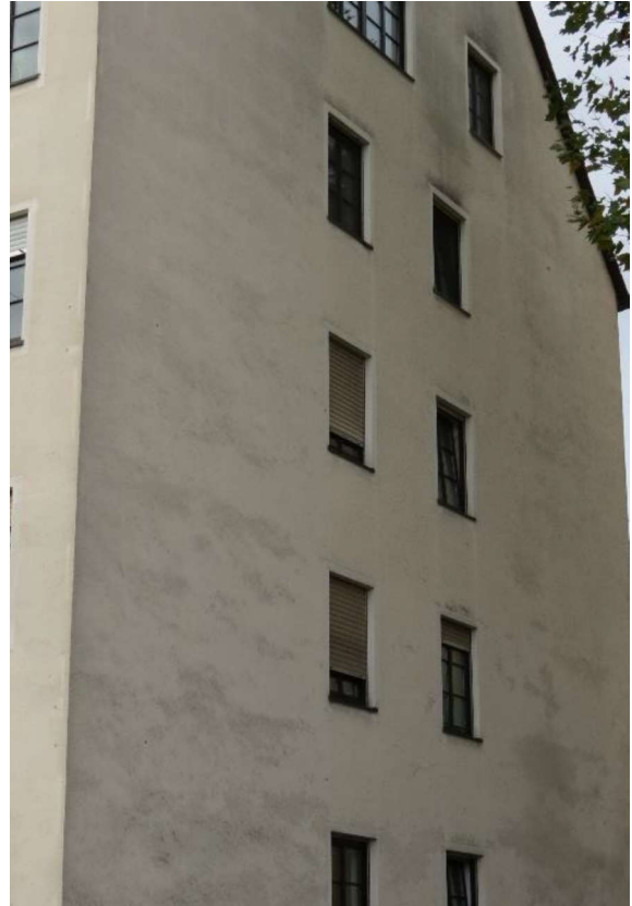
Figure 7: East side of object 96 (left in 2014 and right in 2022) with algae formation and slight rippling at the insulation panel joints. (The rippling is not caused by cavities in the plaster but by unevenness in the plaster layer that is recognizable by the different graying.).
