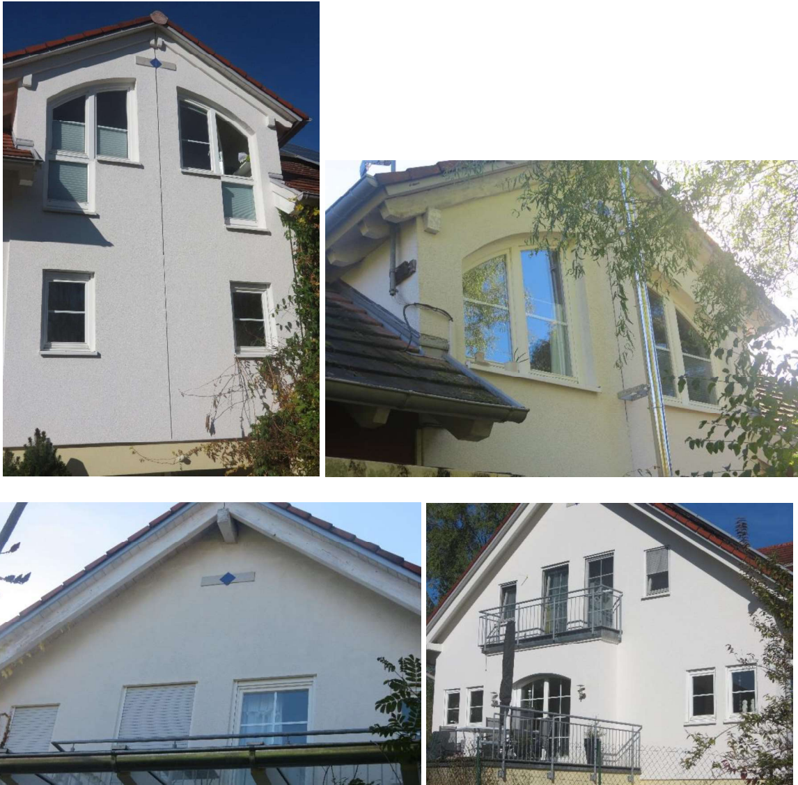
Figure 57: Views of the façades of object 13. Top left: south-east façade - painted in 2020. Top right: north-west façade - only western half painted in 2020. Bottom left: north - east façade. Bottom right: south-west façade - painted in 2020.
