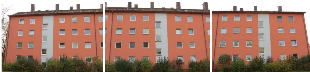
Figure 46: East views of the housing block house numbers 73–77.
