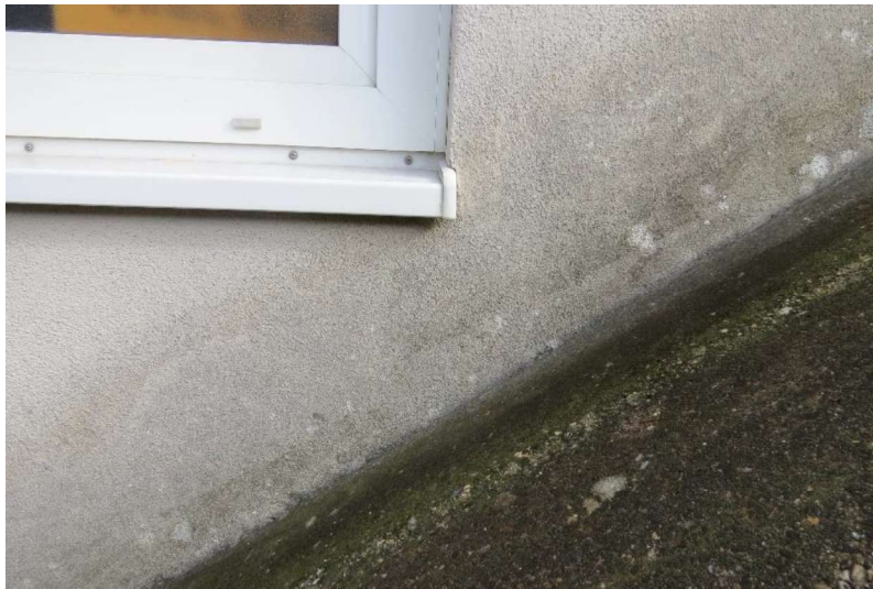
Figure 37: View of the base area of the west façade at the stairs going down, which is insulated with purenotherm.
