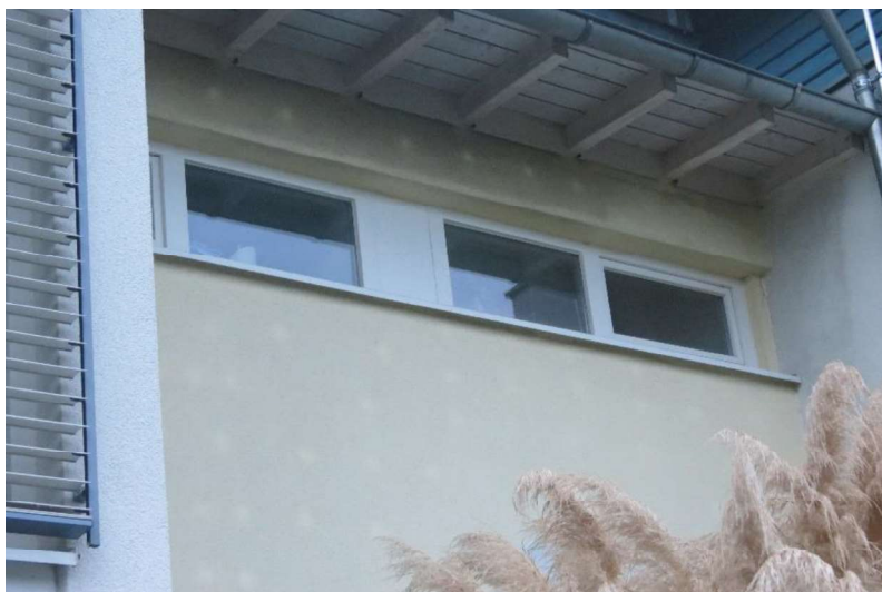
Figure 52: View of the south-east façade of object 9, which is offset to the rear.
