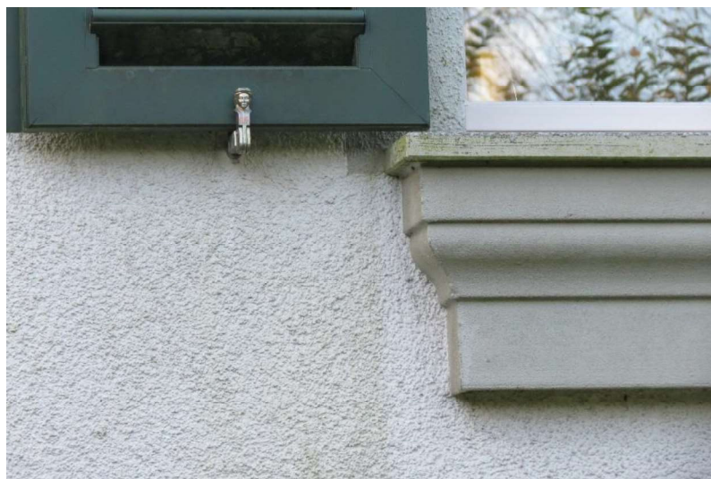
Figure 44: Close-up of a window connection with a frieze on the NW façade.
