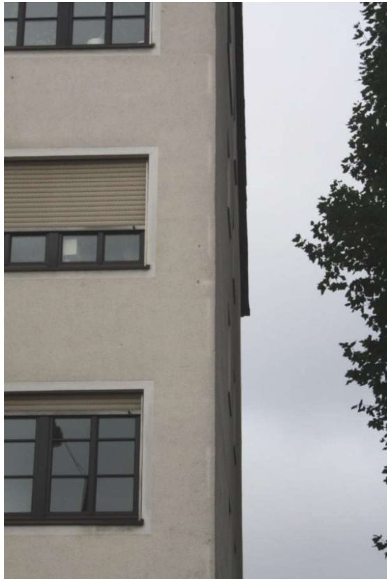
Figure 8: South-east corner of object 96 with appearance of the insulation panel joints through color differences (hardly visible from a distance). Left: View in 2014. Right: View in 2022.
