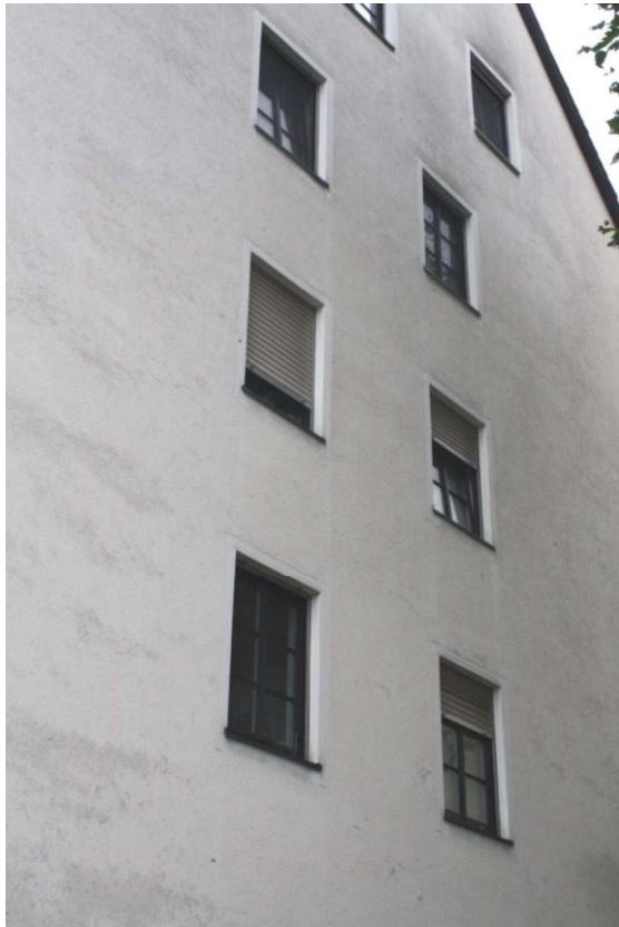
Figure 7: East side of object 96 (left in 2014 and right in 2022) with algae formation and slight rippling at the insulation panel joints. (The rippling is not caused by cavities in the plaster but by unevenness in the plaster layer that is recognizable by the different graying.).
