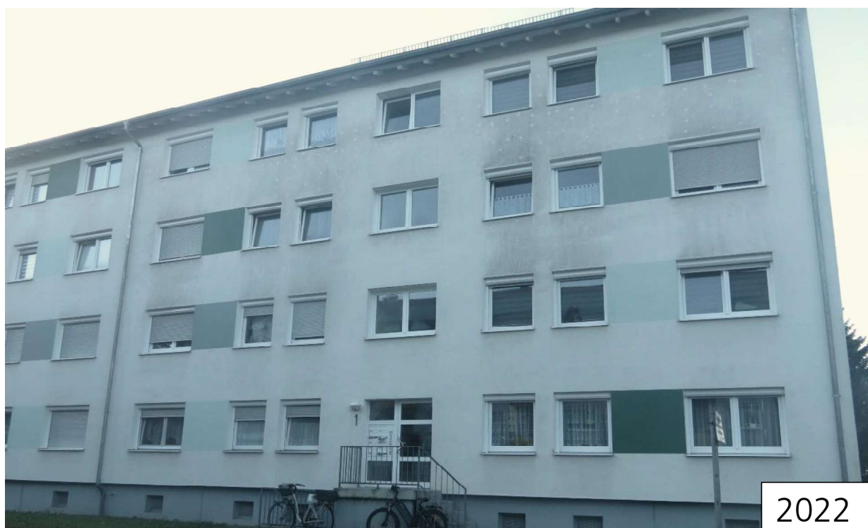
Figure 25: View of the north façade of object 32 (Ebertstr. 1–7, Geislingen a. d. Steige) in October 2022.
