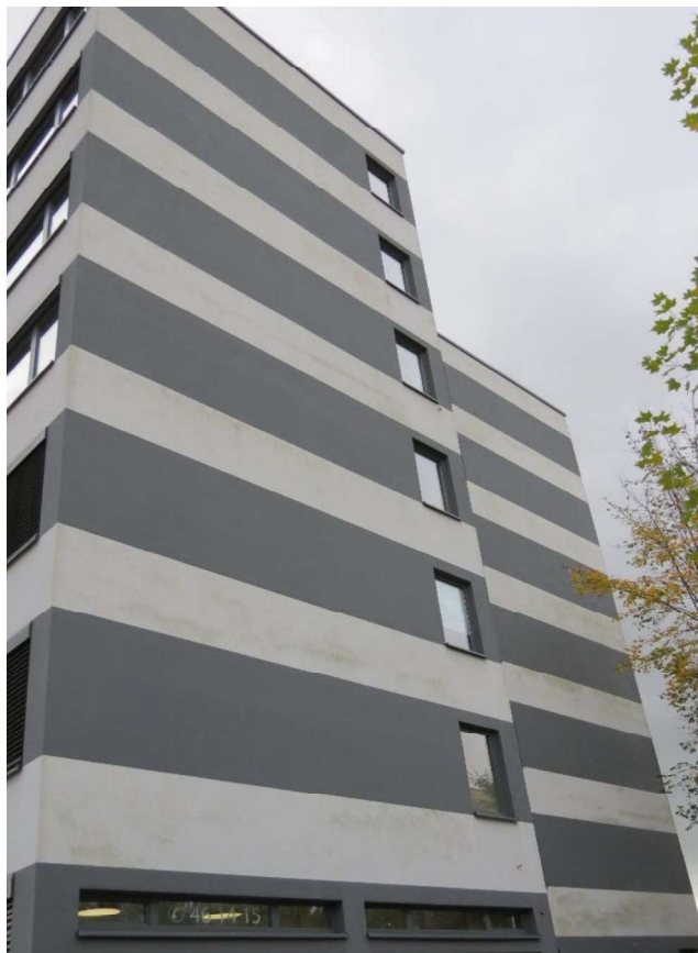
Figure 19: North façade of object 54 in Neumarkt in 2022 with noticeable greening in the white façade areas.
